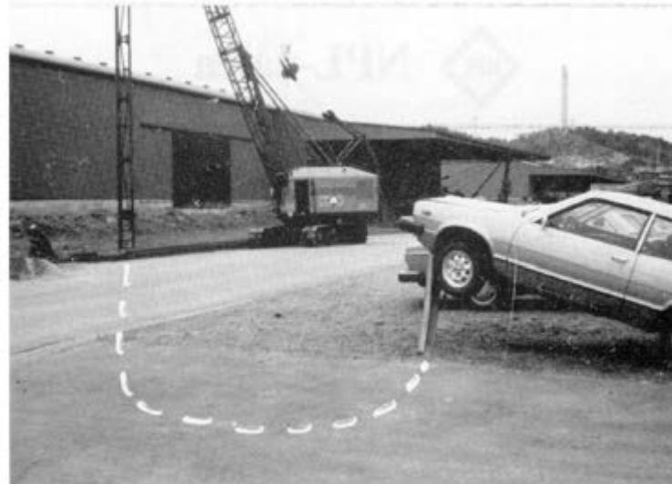
Fig. 2 Side view of car with piling rig in background
